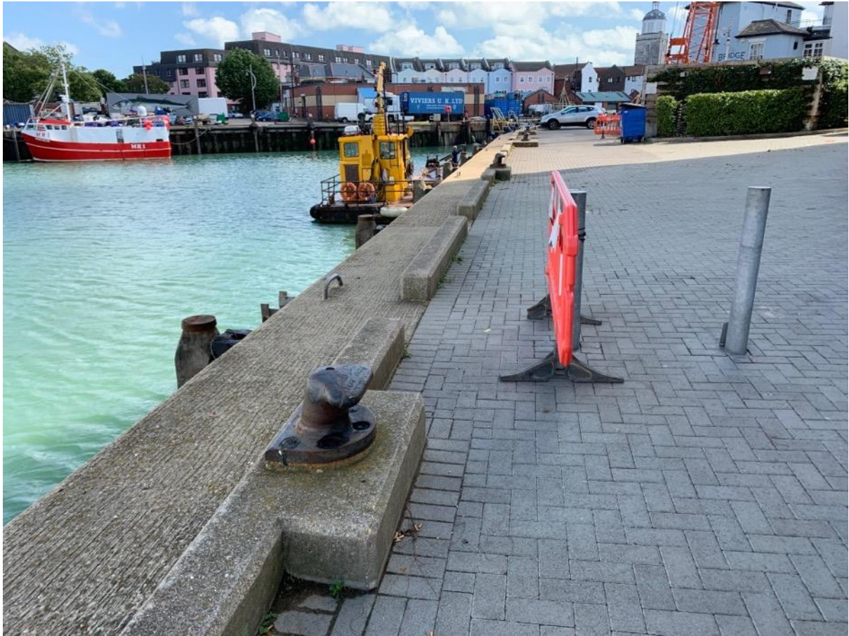
Photograph 6 The Camber Area 2
